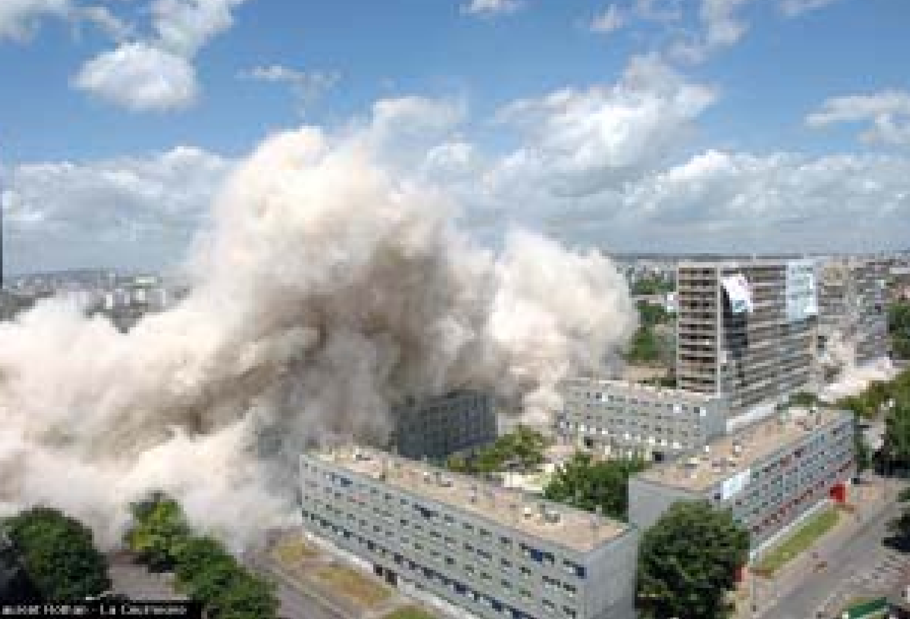
Demolition of Ravel and Presov Buildings, 2004
